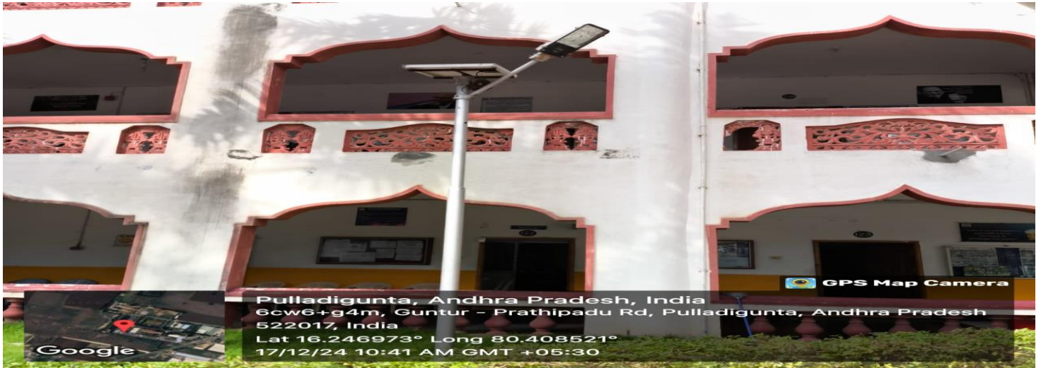
Sensor Based Solar Light in the college campus
