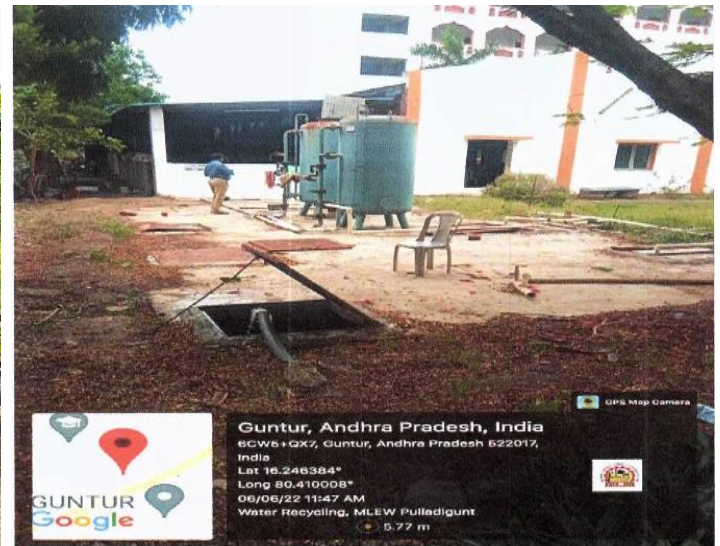
Pit for collection and filtration of waste water from food mess
